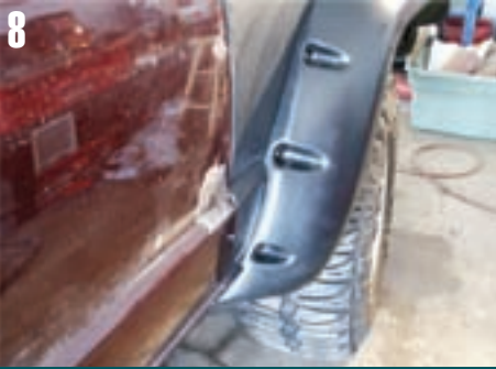
8 Be aware that there is still a rubber gasket to install between the flares and the body. Also be aware that I used sheetmetal screws to temporarily hold these flares and that they will not be permanently attached until I have painted both the flares and the truck.
