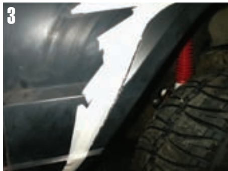
My first cut was with my air grinder. As you can see in the photo, I have cut through the fender in the area that has the support bracket behind. I did this because I would have had a hell of a time cutting through both layers of metal with either the jigsaw or the reciprocating saw.
